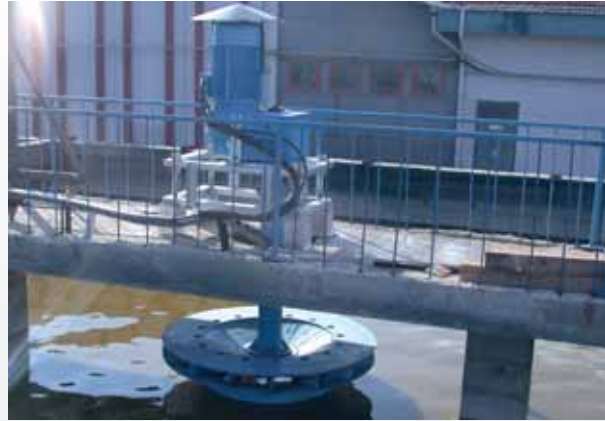
→ 2. Redüktörlü Sabit Tip Aeratör 2. Fixed Surface Aerators with Low and Medium Speed
