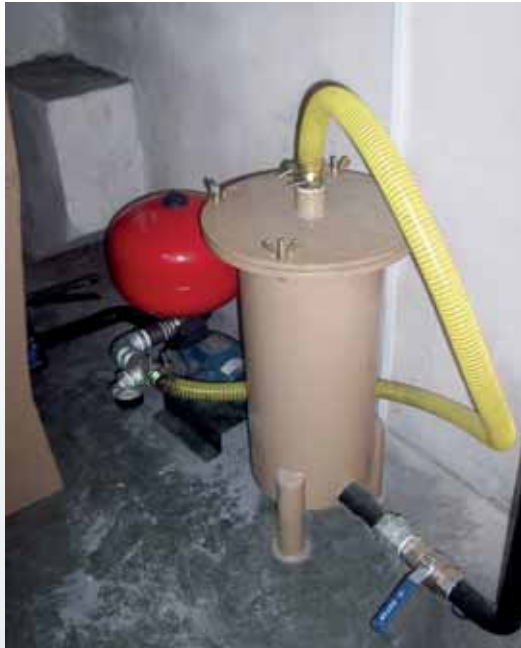
→ 2. Basınçlı Torba Filtreler 2. Pressurized Bag Filters
