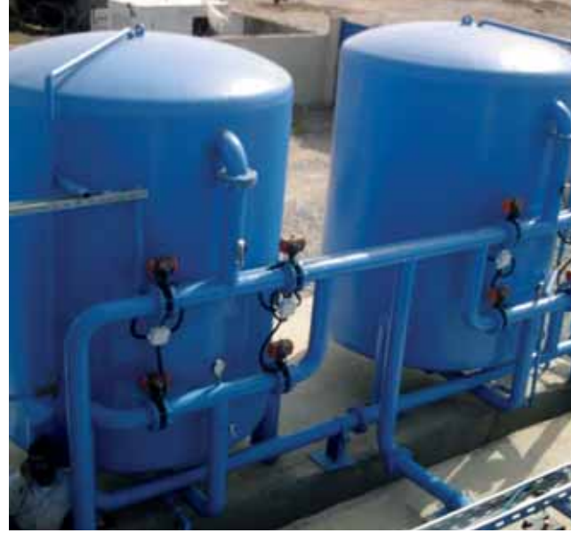
→ 1. MMF ve AC Filtreler / 1. MMF and AC Filters
